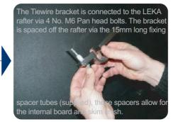
The bracket must be fitted to the LEKA rafter via the fixing plate that is secured within the cavity of the rafter. This plate is not part of the Tiewire kit but comes either pre-fitted to the rafter or loose with the roof ancillaries.
