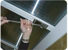
Keeping the wire terminal, tensioner and bracket stud in-line, continue to turn the tensioner until the slack is removed from the wire. DO NOT allow the wire to rotate during this procedure.
