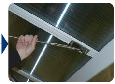
Final tension is achieved once the wire is straight and taut. Do not overtighten and allow the sides of the roof to become distorted. Tighten the locknuts against both ends of the tensioner body.
