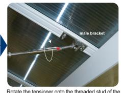
male bracket, this will simultaneously draw in the terminal on the end of the wire. DO NOT allow the wire to rotate during this procedure
